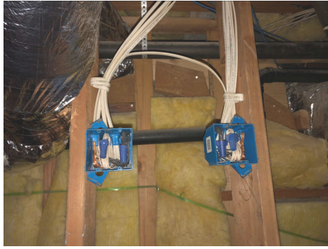
Basement utility room
