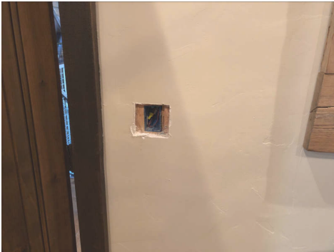
2nd Floor South Bedroom
