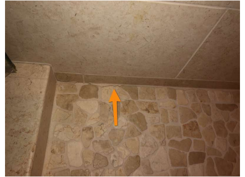
2nd Floor Northwest Bathroom, floor to wall intersection.
