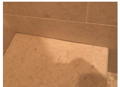
1st Floor Southeast Bathroom
