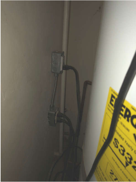
Basement Utility Room
