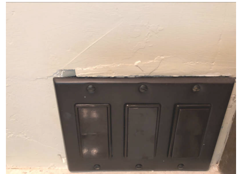
1st Floor Southwest Bathroom
