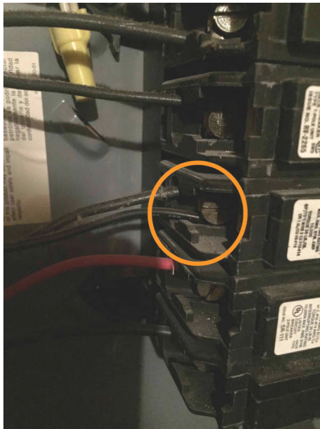
Double tapped breaker
