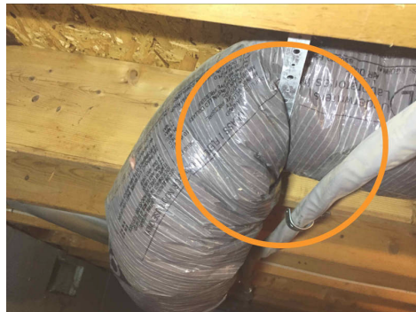
Restriction to airflow. Crawlspace
