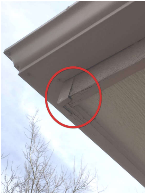
Minor cracking on upper level fascia on the north east corner of the roof.
