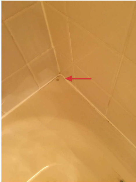
2nd Floor Bathroom Tub
