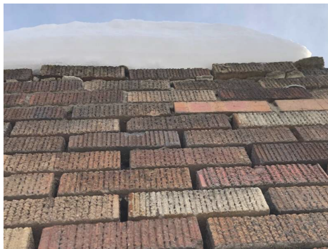
From the top down there are at least 13 courses of brick that need mortar repointed.
