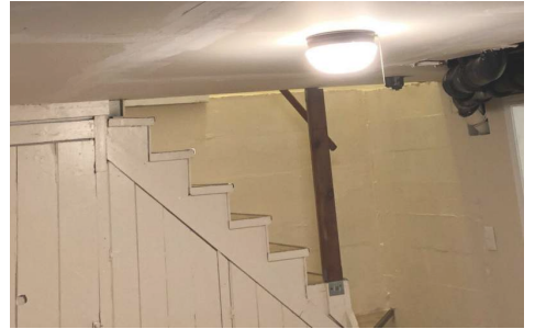
Stairs have no balusters.
