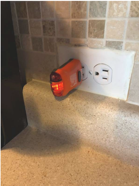
Open Ground/No GFCI.
