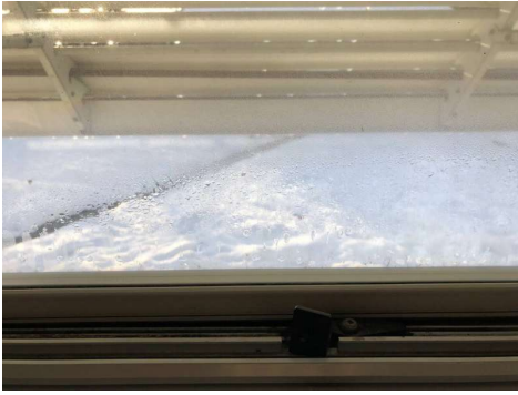
Condensation between window panes.
