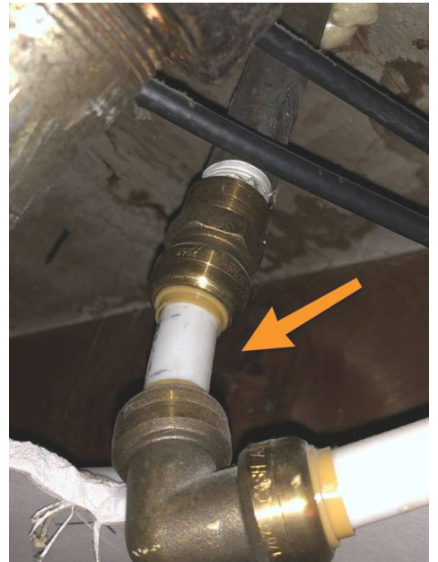
This connection should be made more in-line so that the connection is not under stress.
