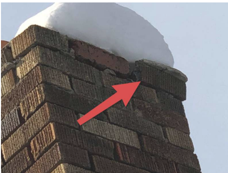
This brick is loose and will fall eventually unless repairs are made.
