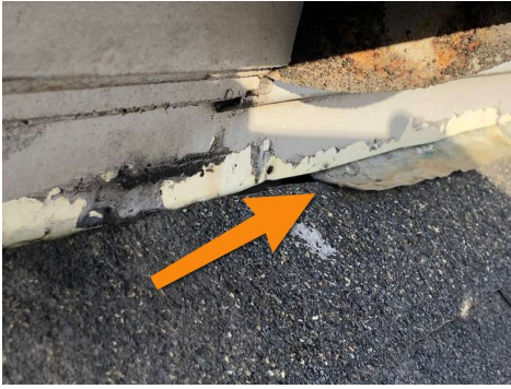
Flashing from sidewall over side entry roof stops short, it should be continuous across roof.
