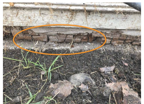
This is classic wood rot that needs replacement with pressure treated wood and the underlying moisture needs to be resolved with better grading and or addition of a window well.
