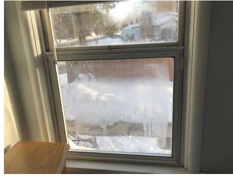
Seals blown between panes.
