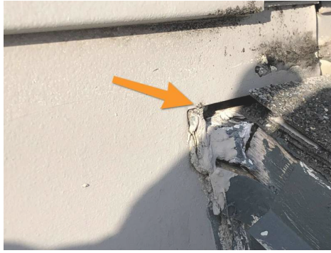
Kickout flashing missing here, with evidence of previous moisture exposure.
