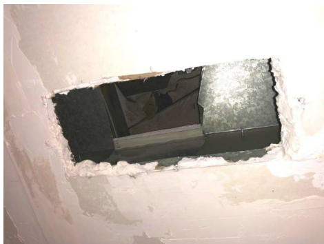
Open ducting above ceiling register.
