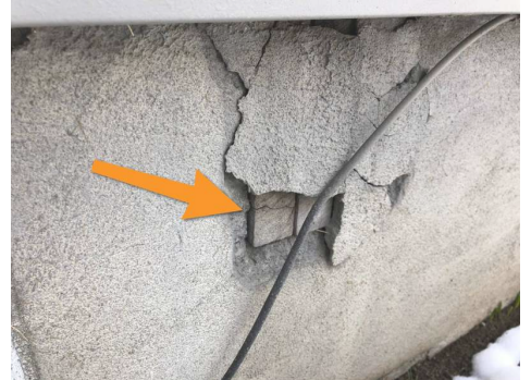
Foundation parge coat is failing. Structural members can be seen. this needs to be sealed up to prevent moisture intrusion.
