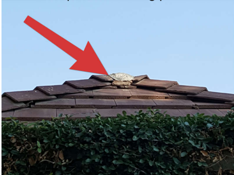
Front (broken / loose)
