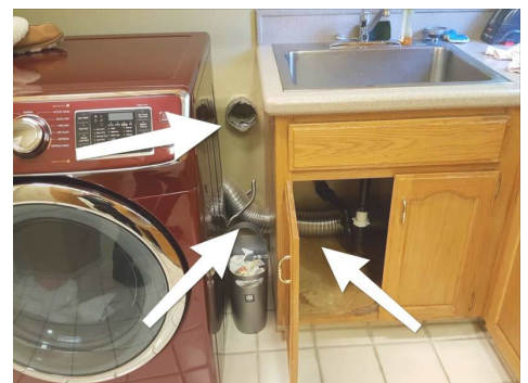
Clean upper vent if upper vent is going to be connected to the dryer
