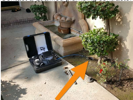
SewerScan started at the clean-out located at the left side of garage
