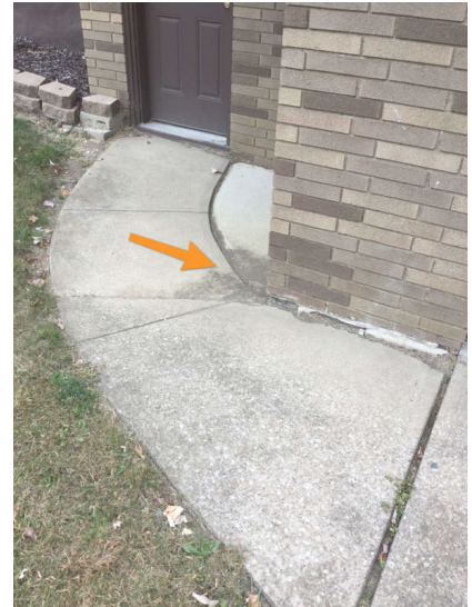
Dirt buildup from water runoff
