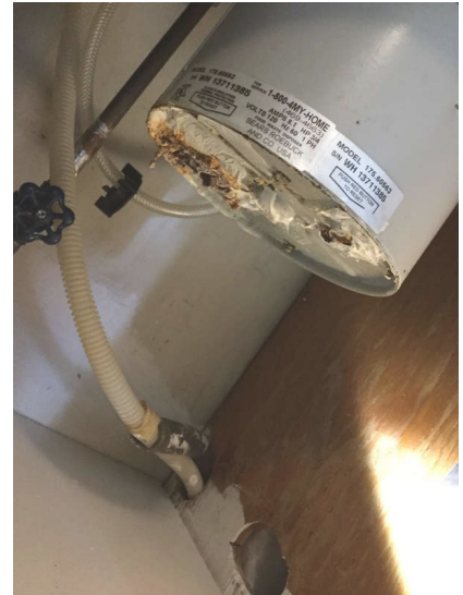
Bottom of unit is corroded and power is disconnected
