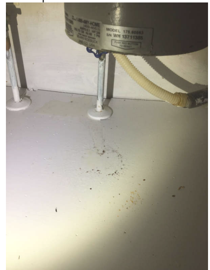
Bottom of unit is corroded and power is disconnected
