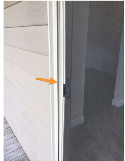
Back screen door damaged.
