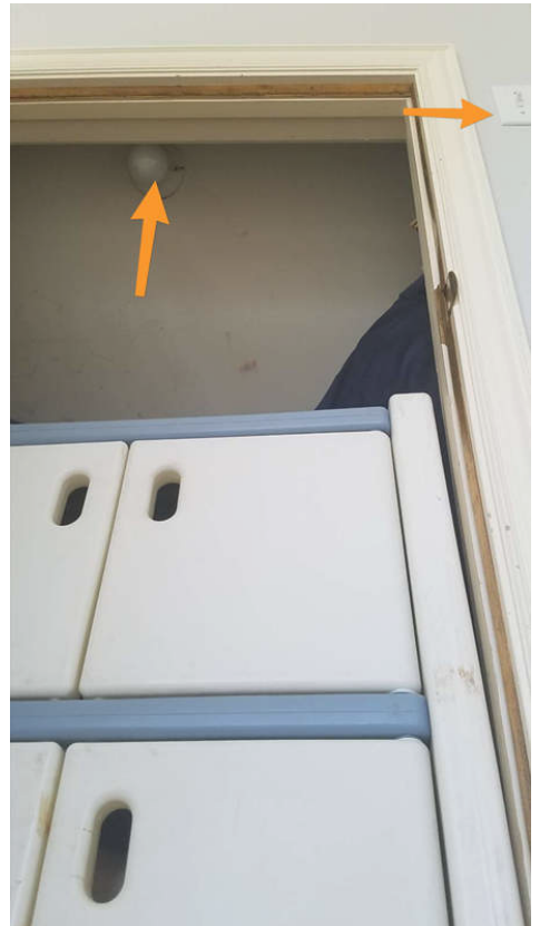
Upstairs Garage apt Closet
