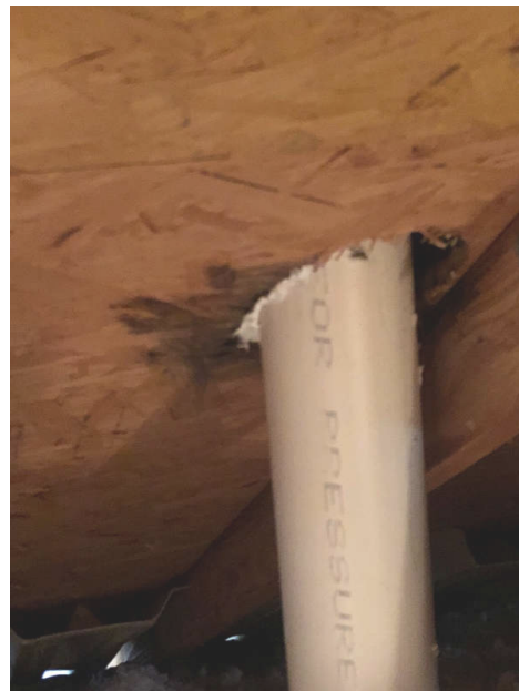
Around vent pipe
