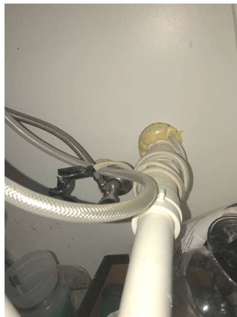
Wire taped off and in reach
