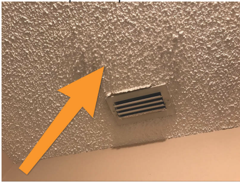
UNIT 1 West Bathroom
