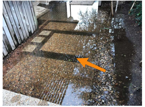
Between Unit 3 and Unit 4
