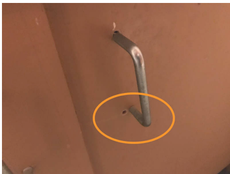
UNIT 2 main office Bathroom
