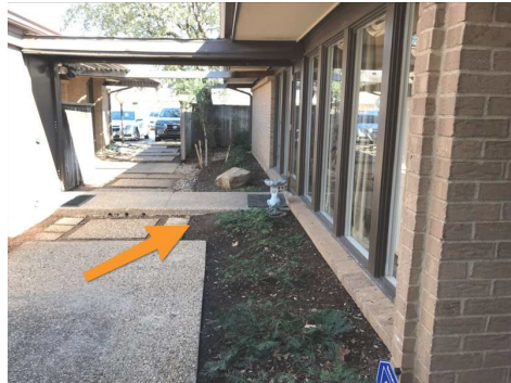
Unit 3 facing North
