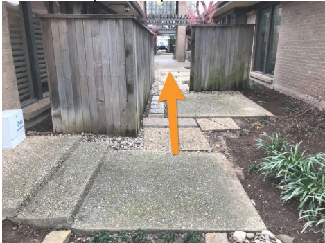
Between Unit 1 and 3
