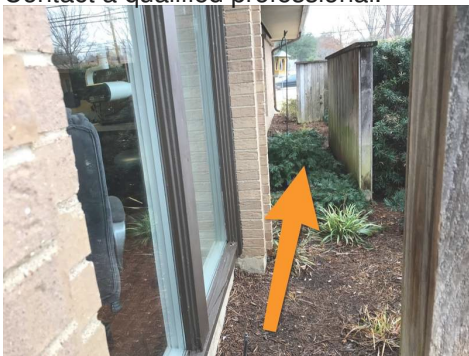
Unit 1 and Unit 4 facing North
