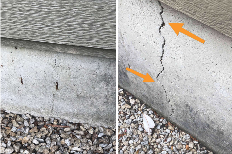
Left front, near elec meter
