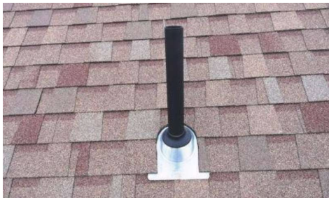
Example of properly flashed DWV Pipe.
