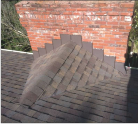
Example #1 of properly flashed cricket.
