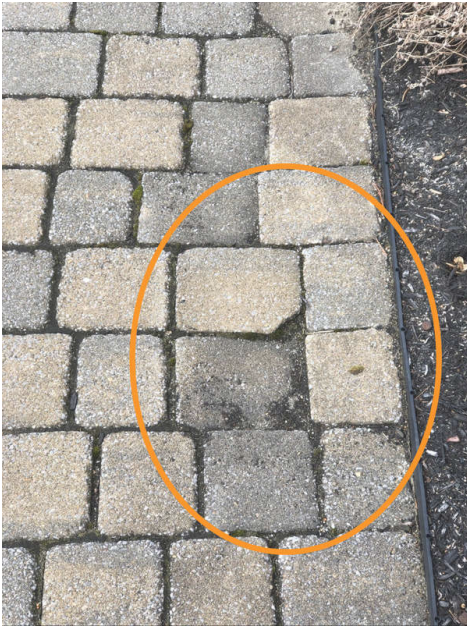
Pavers have sunk along stair tread
