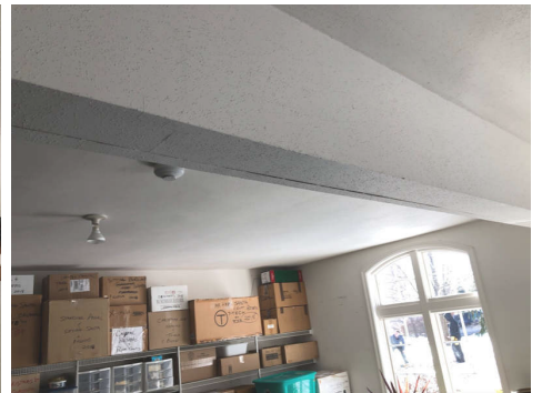
Corner bead pulling away
