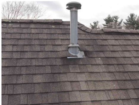
Example of properly flashed DWV Pipe.
