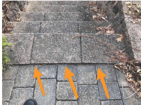
Pavers have sunk along stair tread
