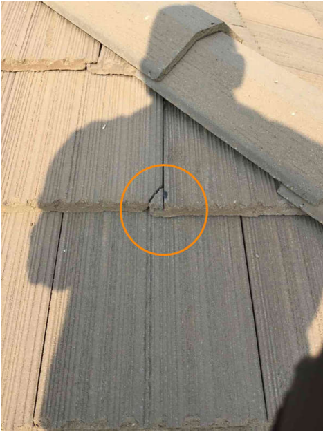
Condition observed at multiple locations.
