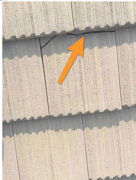
West side of garage roof.
