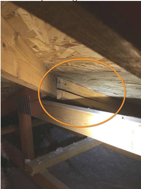
Near end of equipment platform looking Southwest.
