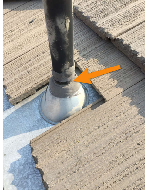
Condition observed at multiple locations.
