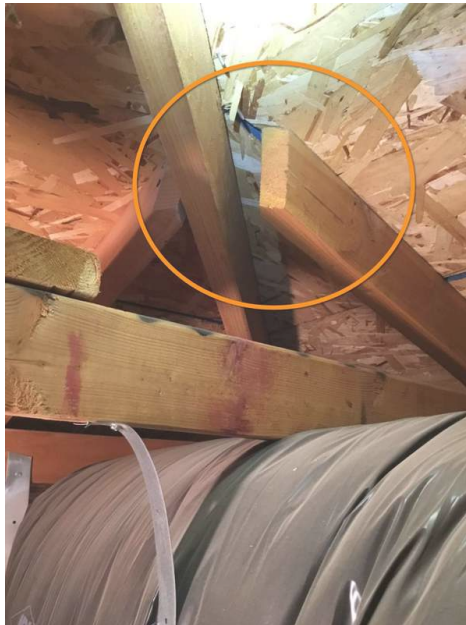
Near HVAC equipment looking North.
