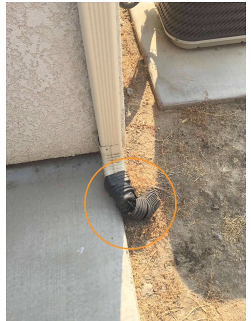
Southwest corner of building.
