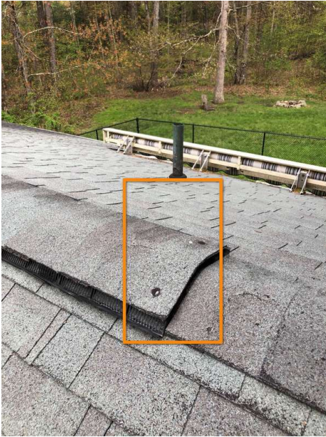
Cracking at ridge vent
