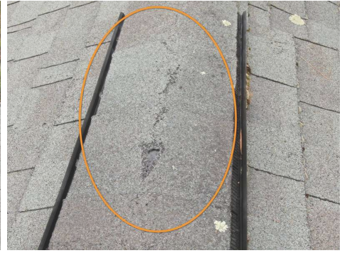
Shingle worn through
