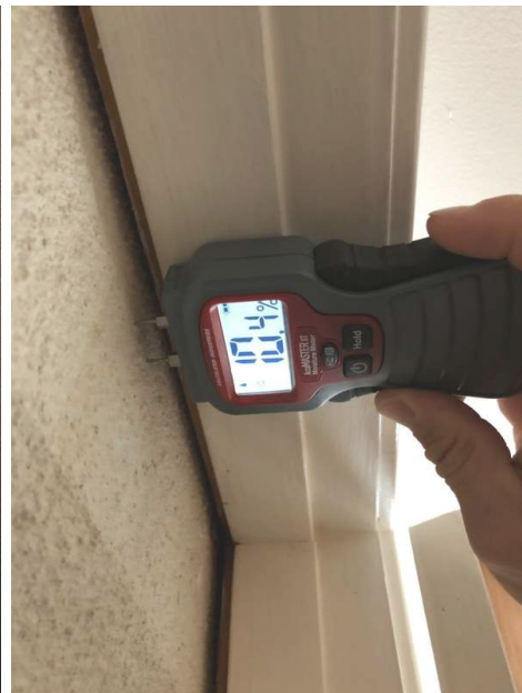
Front Bedroom Closet. 10.4% is consider low on the moisture meter scale. Low: 1.5% - 16% Med: 17% - 19% High: 20% - 33%
