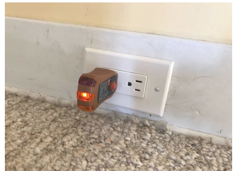
2nd Floor Hallway
