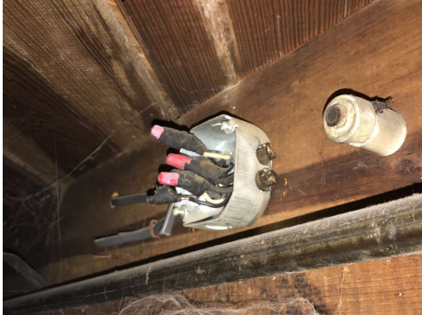
Basement Mechanical Room
