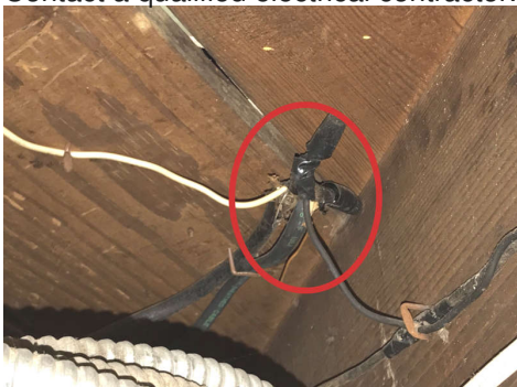
Rec Room - Above Main Beam
