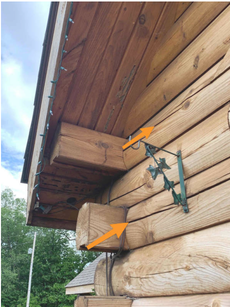
Checking of lumber observed on exterior siding. This is normal as material ages recommend applying
