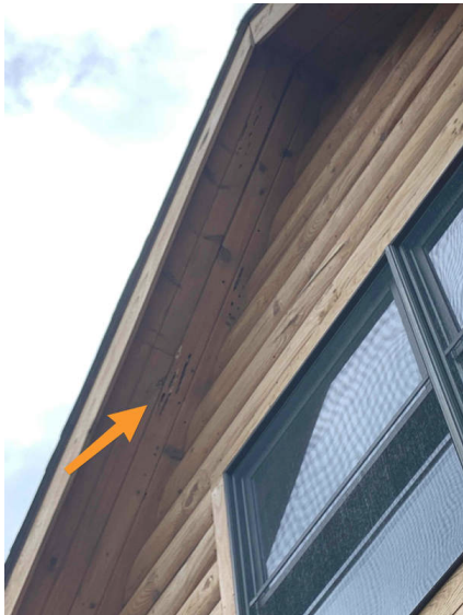
Carpenter bee type damage
