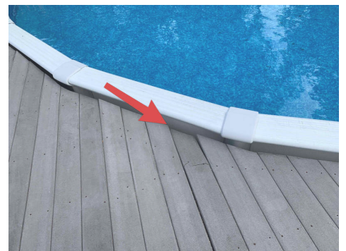
Composite deck board near pool is damaged this is a potential trip hazard
