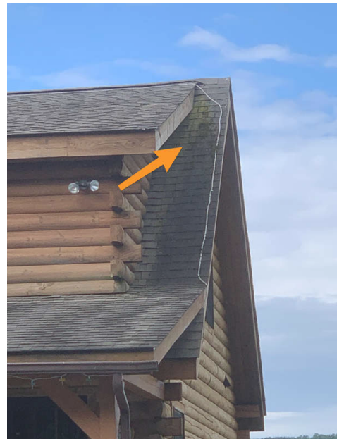
Moss observed on roof surface, recommend cleaning to prevent premature failure of roof material
