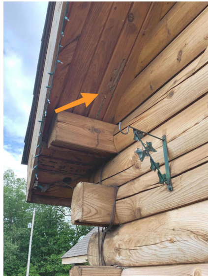
Carpenter bee type damage
