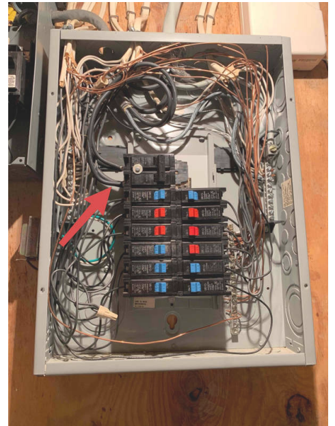
Circuit breaker manufacture prohibits double tapping of this model
