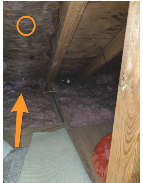
Arrow- Missing baffles Circle - Evidence of condensation (Water stains)
