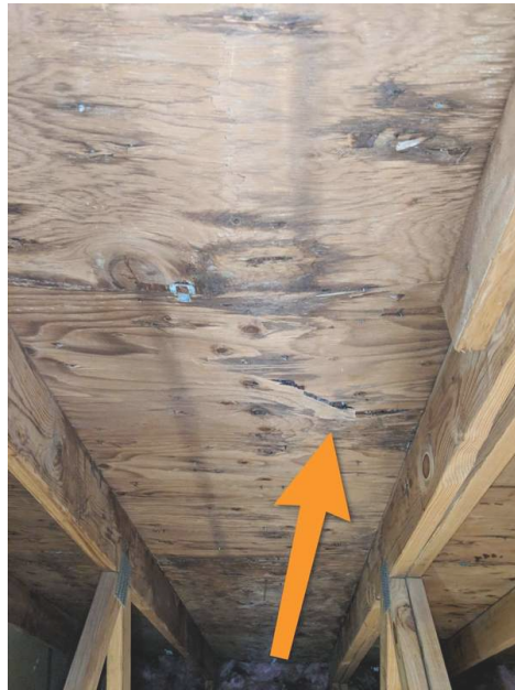
Cracked Sheathing
