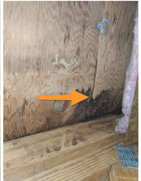
Cracked Sheathing
