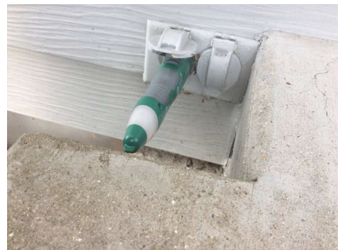
Not GFCI ProtectedWest Exterior
