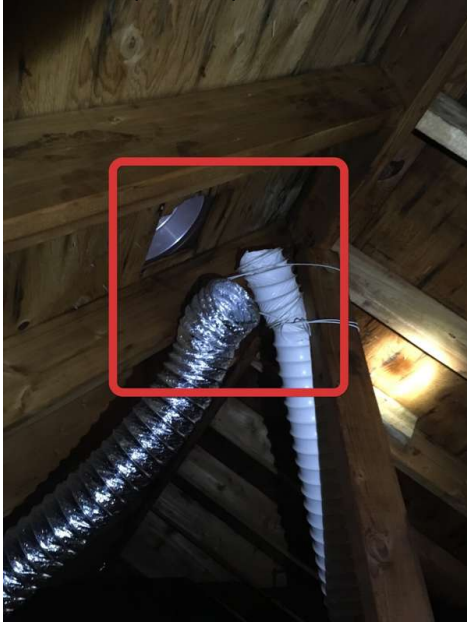
Bathroom Fans Exhausted to Attic
