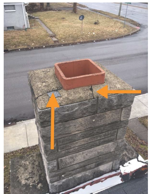
Cracked Chimney Cap
