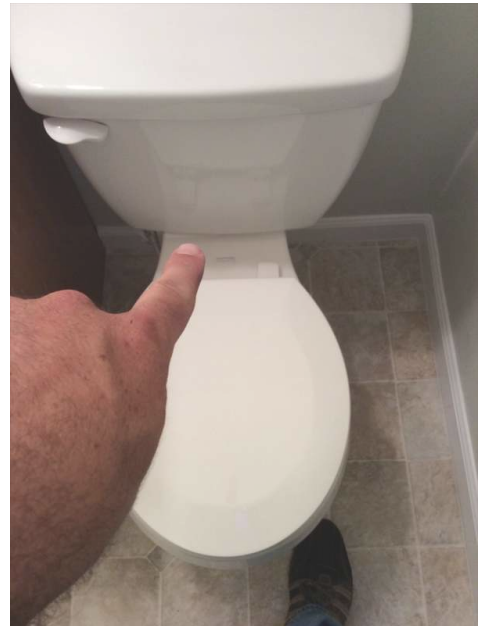
Toilet LooseDownstairs Half Bathroom
