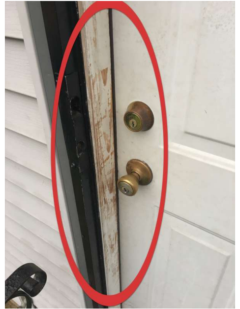
Deteriorating/Missing PaintGarage Exterior Door
