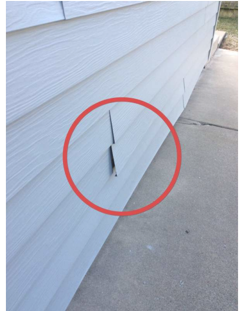
Loose Vinyl Siding West Exterior
