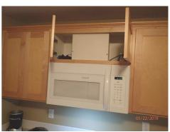
The diverter plate needs to be removed or adjusted to allow for use of the exterior venting.
