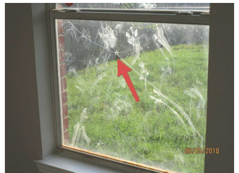
Glass is cracked in window (Southwest bedroom)
