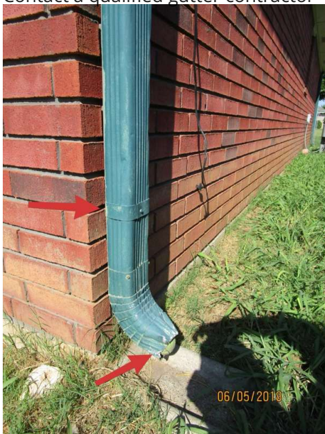
Downspout not secured properly, damaged, and plugged. (Southwest corner of home)
