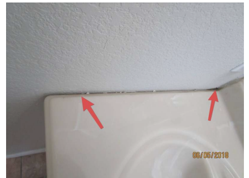
Gap between wall and sink in master bathroom.
