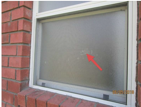
Multiple screens have holes in them (this is on North side of home)
