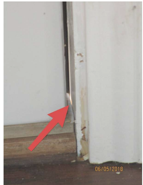
Noticeable gap on bottom (right) of back door.
