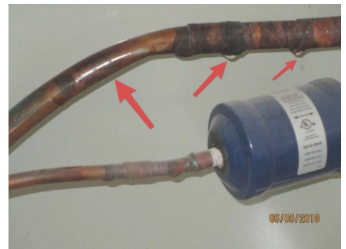
Insulation missing from Suction line, and line is "sweating." (this photo taken in HVAC closet on inside of
