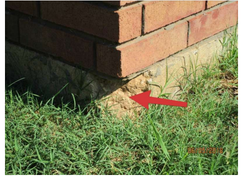
Foundation on both Southwest and Northwest corners of home chipping away, commonly called "Corner Pops."
