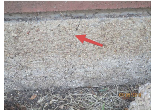
Multiple minor cracks in foundation (North side of home)
