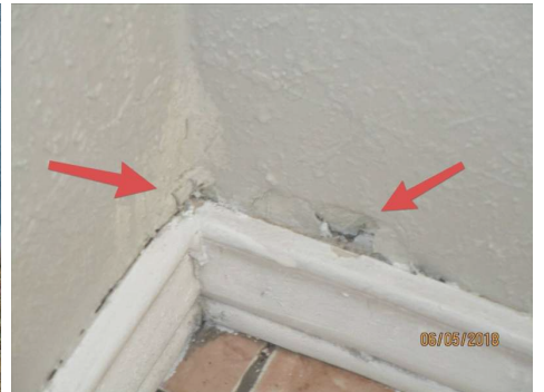
Drywall shows signs of previous water damage (master bedroom closet on wall opposite side of sinks)
