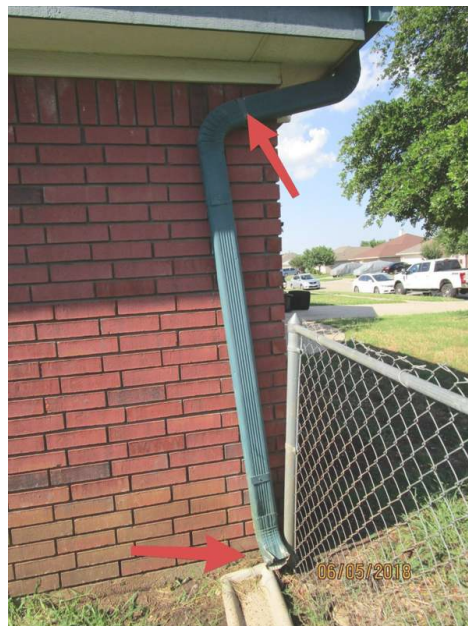
Downspout loose, damaged, and not aligned with splash block. (Southeast corner of home)
