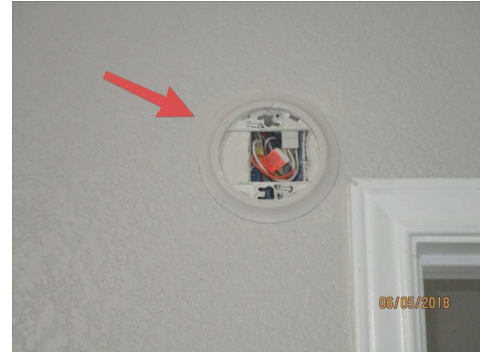
Smoke detector missing (front bedroom to "right" of front door).
