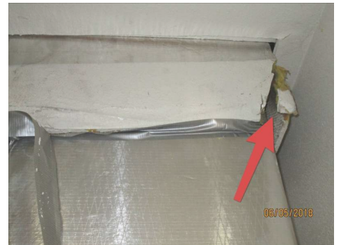
Duct system (above evaporator unit in HVAC closet) not sealed properly.
