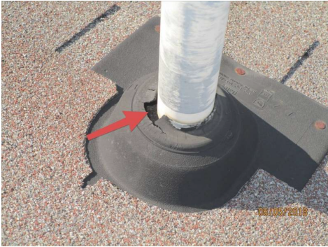
Multiple vent "boots" were deteriorated (South, North, and West sides of home).
