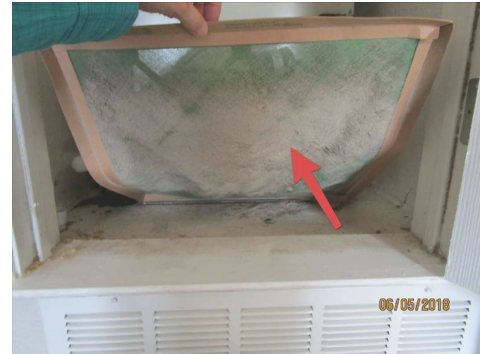
A/C filter dirty and flimsy.
