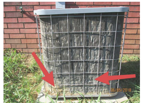
Condenser unit fins in very poor shape.
