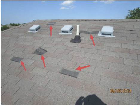
Numerous shingles missing, and other shingles not laying properly. (this pic is on West side of roof facing backyard).
