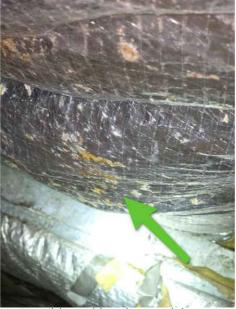
Possible mold at ducts. A lab test may be needed to confirm.
