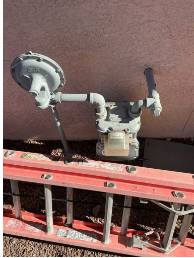
Type of Gas Distribution Piping Material: Black Steel Comments:
