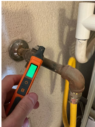
Type of Gas Distribution Piping Material: Black Steel Comments:
