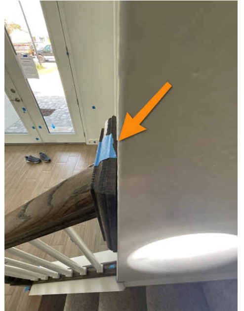
Staircase Handrails (Gap)
