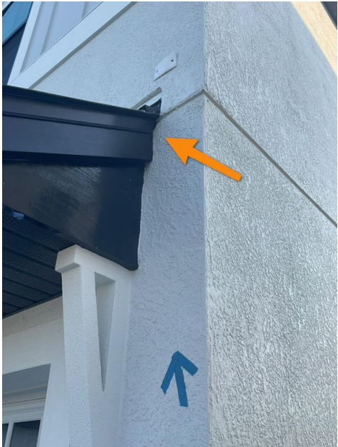
Front Elevation Gaps
