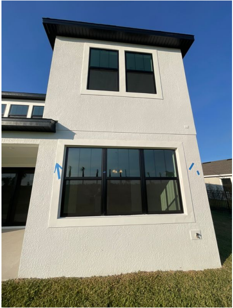
Back Elevation Missing Paint
