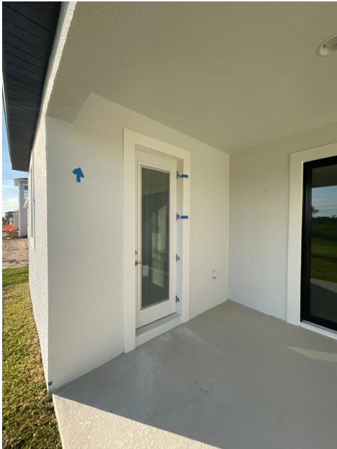
Back Elevation Missing Paint
