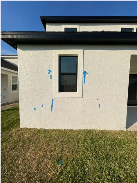
Back Elevation Missing Paint
