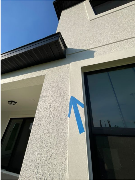
Back Elevation Missing Paint
