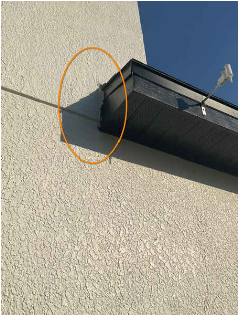
Right Elevation Missing Paint
