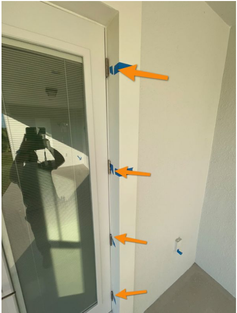
Back Elevation Entry Door (Gaps)
