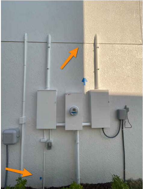
Right Elevation Missing Paint
